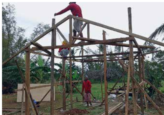
Muslim Aid supports the construction of shelter. Photo: Muslim Aid
