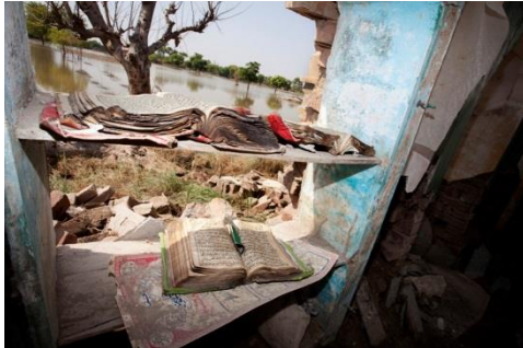
Mosque damage from floods, Subzu Jat Punjab, Pakistan
